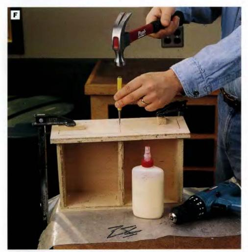
PHOTO F: Install the drawer front on the drawer carcase with glue and finish nails. Note that the front overhangs the drawer carcase  $\frac{5}{8}$  in. on the sides and  $\frac{1}{2}$  in. on the top and bottom.
