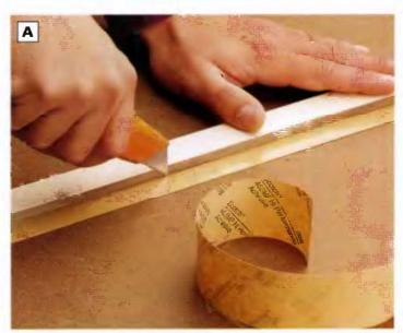
PHOTO A: Peel off the protective paper that covers the adhesive backing of the maple veneer and adhere it to the ¼-in.-thick walnut strips. Trim the veneer to fit the walnut with a sharp utility knife.
