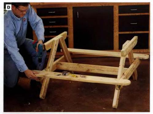
PHOTO D: Set the frame upright on the floor to secure the seats into position. The ends of the seats should overhang the seat stringers by about  $4\frac{1}{2}$  In. Make the outside edges of the seats overhang the ends of the seat stringers by 1 In.
