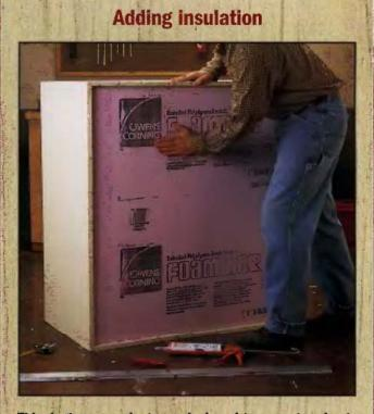
This doghouse project was designed to accept a sheet of 1-in.-thick rigid foam insulation below the bottom panel. Rigid foam is a good choice because it is relatively inexpensive and unaffected by ground moisture. Measure and cut the insulation with a utility knife. Glue it in place with construction adhesive.
