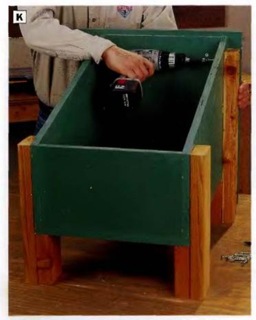
PHOTO K: Install the leg assemblies to the cart box with  $1^{1/2}$ -in. screws. The front legs should butt against the back of the cart face. Attach the rear legs so they are flush with the cart back.
