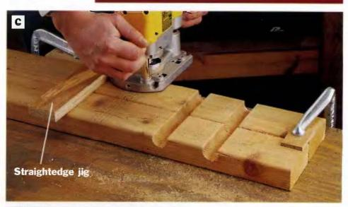
PHOTO C: Gang-rout notches in the back supports to ensure that the notches will line up perfectly on both pieces. Use a <sup>3</sup>/<sub>4</sub>-in. core box bit, and cut the notches in several passes of increasing depth. We clamped a short T-square style straightedge jig to gulde the router when cutting.
