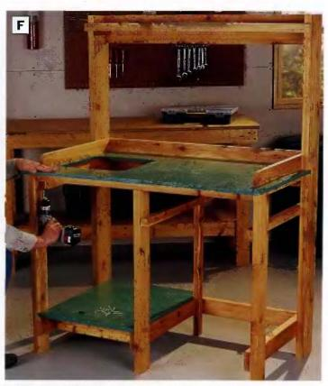
PHOTO F: Install the back splash and slde splash pieces on the countertop, then fasten the countertop to the bench framework by driving screws through the stretchers from below and Into the countertop.
