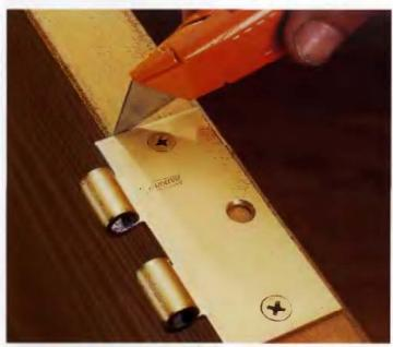
Remove the hinge pin (if its removable) and position the hinge leaf or strike plate on the edge of the door or on the door jamb. Tack it into place with screws, then score an outline around the plate with a utility knife. This prevents the wood from splintering past the ends of the mortise.
