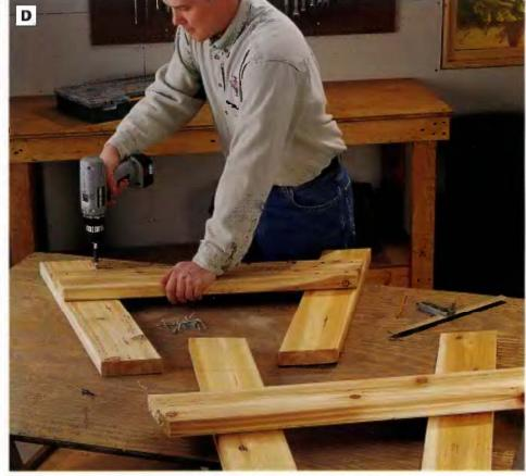
PHOTO D: Cut the legs and leg braces to size, and cut the ends of the parts at 75° angles. Use the *Table End View* drawing, page 397, as a reference for cutting the parts. Then construct the two table leg assemblies by fastening each leg brace to a pair of legs with deck screws.
