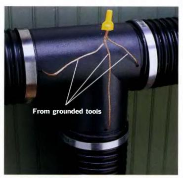
**2** Drill exit holes at hole connectors and pigtail ground whres together with a wire nut. You may need to caulk around the wire openings to maintain the vacuum seal.
