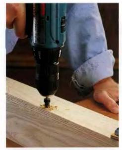
Drill a counterbored pilot hole using a counterboring bit or by drilling a pilot hole, then counterboring for the screw shank and the screw head, according to the dimensions in the chart above.
