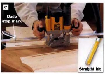
PHOTO C: Rout  $44 \times 14$  in. dadoes along the Inside faces of the sides, 12 in. in from the back edges, using a 14-in. straight bit (See inset photo). Stop the cuts 212 in. from the bottom edges of the sides.
