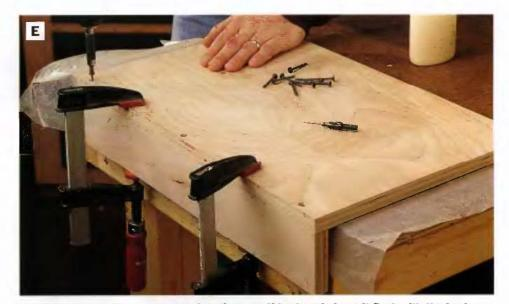
PHOTO E: Spread giue along one edge of the sheif back and clamp it flush with the back edge of the sheif. Attach the parts with countersunk 2-in. drywail screws.
