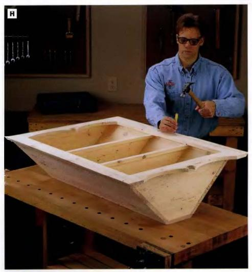
PHOTO H: Attach the face frame to the cupboard carcase with give and 4d finish nalls. Drive the nallheads below the face frame surface with a nailset.
