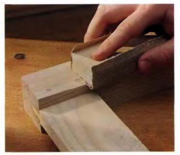
Finally, remove any excess glue with a scraper and sand the surface smooth with sandpaper and a wooden sanding block.
