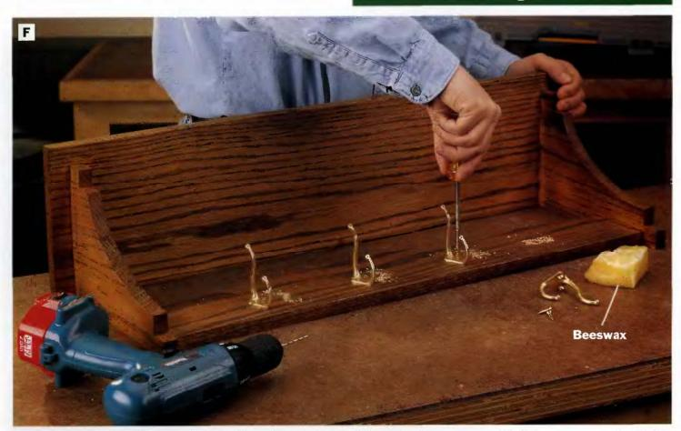
PHOTO F: Lay out and attach four coat hooks to the coatrack back. Drill pilot holes for the screws, especially if the screws are made of brass. Space the hooks about 6 in. apart. Tip: Coat the screw threads with beeswax to make them easier to drive into the oak.
