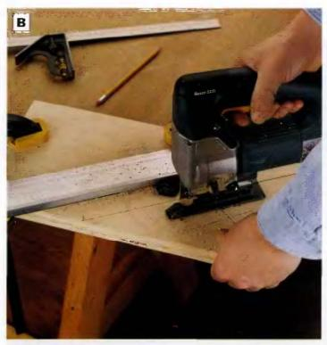
PHOTO B: Lay out and cut the side panels to shape with a jig saw guided by a ciamped straightedge.
