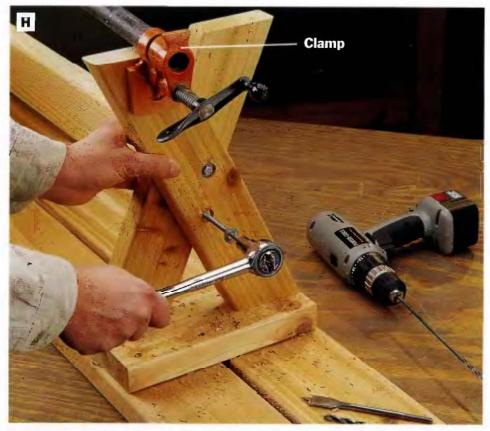
PHOTO H: Cut the bench braces to length and clamp them in position 51/2 ln. from the bottoms of the legs on each bench. Drill 3/4-in.-dla. counterbores in the outermost legs to recess two lag bolt heads, then drill pilot holes through the counterbored holes to install the lag bolts. Sllp a washer onto each lag bolt before you screw it through the legs and into the bench braces.
