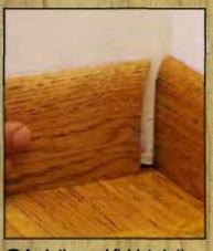
3 Apply the wood finish to both boards, then slip the beveled board into the corner so it overlaps the end of the square-cut board.
