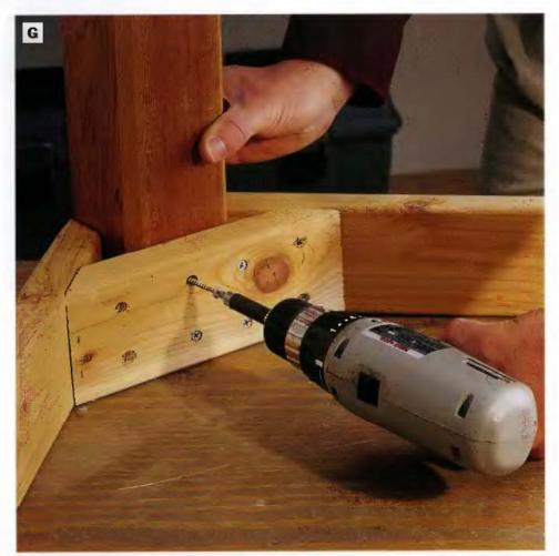
PHOTO G: Assemble the table legs, aprons and corner braces. Attach the parts by driving  $2^{1}/2$ -in. galvanized deck screws through countersunk pilot holes in the leg braces. Fasten the brace to each apron with a pair of screws driven in at an angle into the aprons, and use four screws for securing the leg. Be sure the legs are tight against the aprons and braces as you drive the screws.
