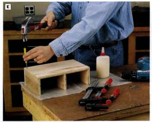
PHOTO E: Fasten the drawer sides and divider to the bottom and back with the drawer arranged upside down on your bench. Giue, ciamp and nail these joints.
