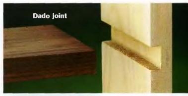
DADO & RABBET JOINTS interlock to add strength and increase glue surface. There are many variations of the joint, including the dado joint, (above) the rabbet joint (page 65, top left) and the combination dado/rabbet joint (page 65, top right).
