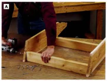
PHOTO A: Attach the back legs to the seat stretchers with 2-in. galvanized deck screws. Countersink the screw heads.
