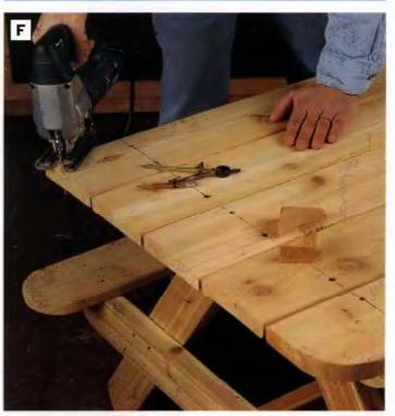
PHOTO F: Mark a 2¾-in. radius on each of the four corners of the tabletop, and trim the corners with a jig saw.
