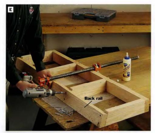
PHOTO E: Build the bench frame by installing four struts between the front and back bench rails with give and screws. In this photo, the bench frame is upside down. Notice that the beveled edge of the back rail lines up with the edges of the struts, leaving an offset on the other edge.
