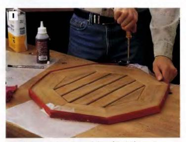
PHOTO I: Glue and clamp the two halves of the tabletop rall assembly together with polyurethane glue and a strap clamp. Cover the glued corners with wax paper. Nail, rather than glue, the slats in place.
