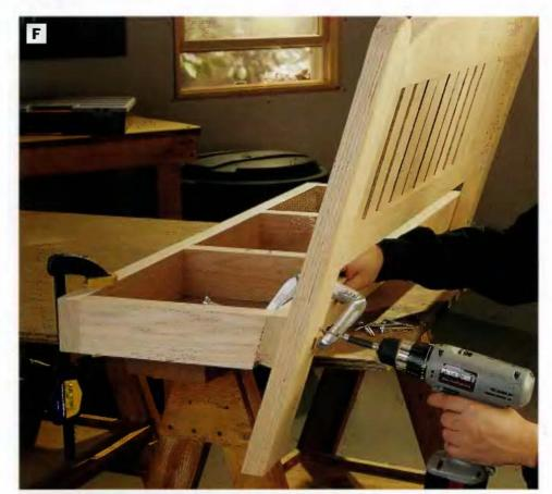
PHOTO F: Fasten the back assembly to the bench frame by driving countersunk screws through the stiles and into the back bench raii. Be sure the bottom beveied ends of the stiles are parallel with the bottom edges of the bench.
