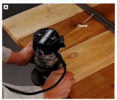
PHOTO A: Clamp the tabletop slats together and rout the ends and edges with a ½-in. roundover bit. Clamping the slats together will produce an even profile on the ends of the slats.
