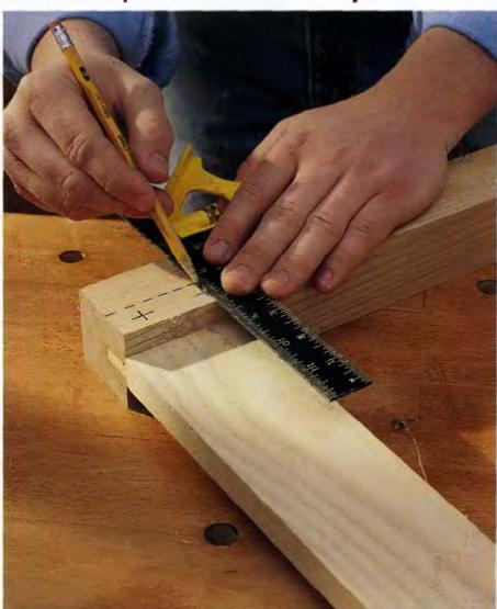
1 Cut the mortises and tenons, then give and ciamp the joint. Let the give set up, then iay out the location of the pins with a pencii and combination square. Use at least two evenly spaced pins for each joint, making sure the guide holes are at least  $\frac{3}{8}$  in. from the edges of the boards.
