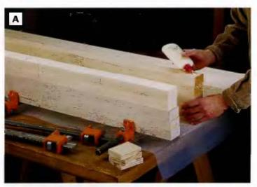
PHOTO A: Face-glue the benchtop in sections of four or five boards, then face-glue the sections together.
