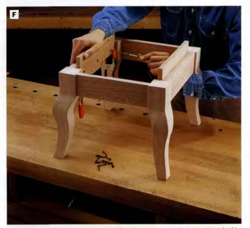
PHOTO F: Hold the base cleats In position with spring clamps so each cleat's rabbet shoulder is flush with the top of the adjoining front or back rail. Drill pilot holes and drive #8  $\times$  1¼-In. flathead wood screws to attach the parts.
