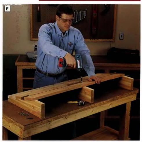
PHOTO E: Attach the back slats along the angled edges of the back supports with screws. Use ¼-in. spacers between the back slats to hold the slats apart.
