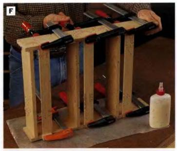
PHOTO F: Dry-fit the front ralls in their notches in the sides. The rails should fit flush with the front edges of the sides. Once they do, glue and clamp the front ralls in the notches.
