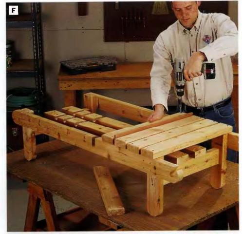
PHOTO F: Screw the five scat slats to the seat rails. Determine and mark the positions of the end slats first, then space the remaining three slats evenly between the end slats. If the slat space is consistent on your chair, use a scrap spacer to make spacing easy when fastening the parts.
