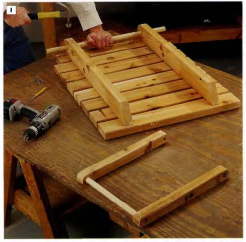
PHOTO I: Tack the back rest dowel in place on the back rest ralls with #6d galvanized finish nails. Drive the nails through the rails and into the dowels. To keep the dowels from splitting, drill a pilot hole for the nails first.
