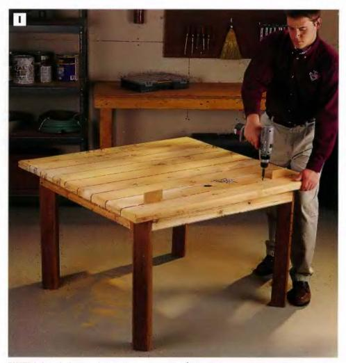
PHOTO I: Attach the top slats to the aprons with 2½-in. deck screws. Fasten the center slat first, then work outward. This way, the overhang will be consistent on both ends of the table, and the slats will be evenly positioned. Use a pair of 3/16-in, spacers to create uniform gaps between the slats.
