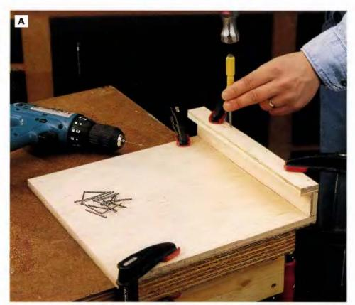
PHOTO A: Assemble the book rest, shelf and shelf lip with glue and 1¼-in. finish nails. Drill pilot holes first for the nails.
