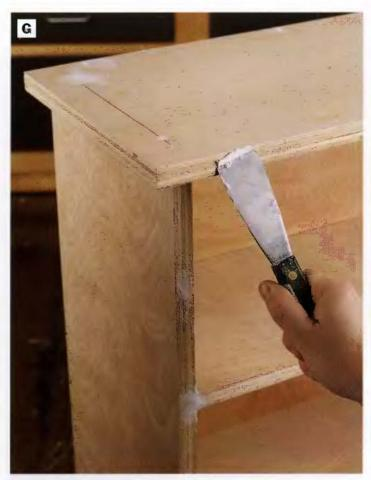
PHOTO G: Conceal the screwheads and any volds or gaps in the plywood with wood putty. Sand the putty smooth when it dries.
