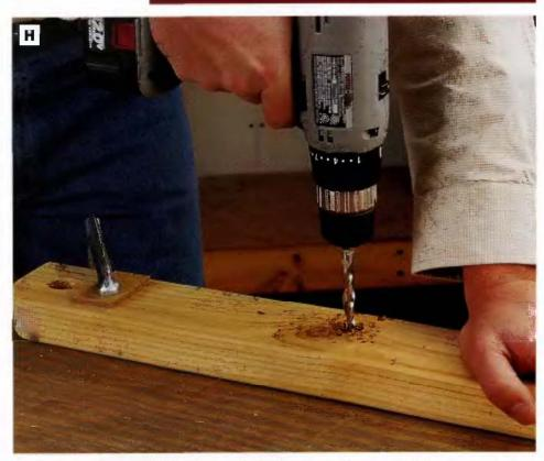
PHOTO H: Drill  $^3$ /8-In.-dia. holes through the back rails, centered on the 1-In.-dia. counterbore holes. These holes will house pivot bolts for the adjustment brace that supports the chair back and holds it in one of three positions.
