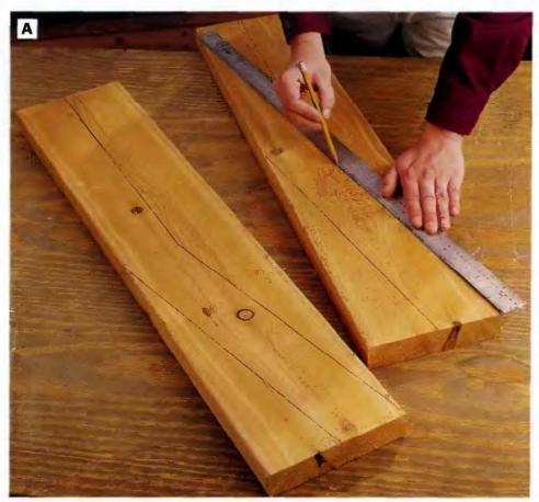
PHOTO A: Lay out and cut eight back chalr legs to shape. Use the Back Legs drawing, page 389, to establish reference points for drawing the leg shapes. Connect the points with a straightedge.
