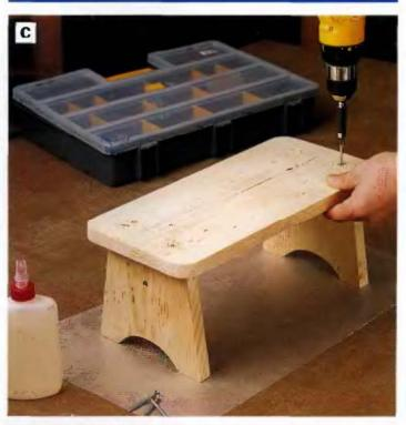
PHOTO C: Attach the top to the stretcher and legs with give and screws. Lay out the stretcher and ieg iocations on the top first, for iocating the screws.
