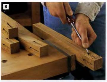
PHOTO K: Drill out the leg mortises on the drill press to 1/2-in. depth. Clean up the waste from the shoulder of the mortises with a chisel.
