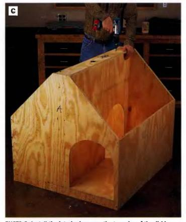
PHOTO C: Install the interior brace on the top edge of the divider and so It Is centered on the short, flat top edges of the doghouse front and back. Fasten the parts with screws.
