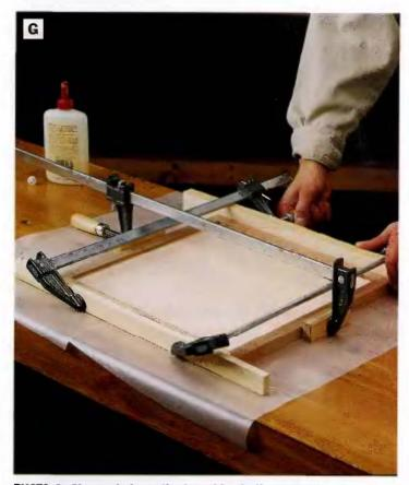
PHOTO G: Glue and clamp the tray sides to the tray bottom, aligning the mitered corners. No additional reinforcement is required.
