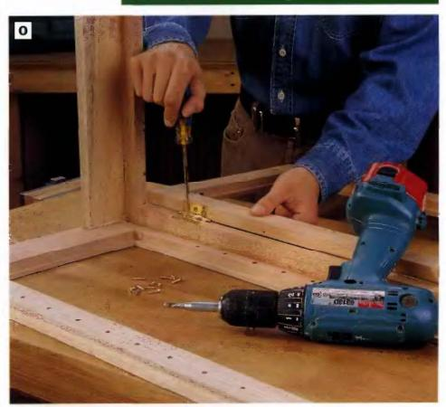
PHOTO O: Cut hinge mortlses into the edge of the face frame stile and attach the door to the cabinet with hinges and screws. Drill pllot holes for the screws to keep them from splitting the wood. Support the door from beneath as you attach the hinges.
