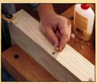
2 Drive the screw, then apply glue to the end of a wood plug and insert it into the counterbore hole.
