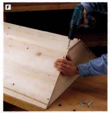
PHOTO F: Assemble the carcase parts using 1½-in. flathead wood screws to reinforce the joints. Attach the cupboard back by driving the screws at an angle through the back and into the sides.
