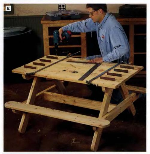
PHOTO E: After setting the slats into position on the top stretchers and marking alignment lines for screw holes, insert spacers between the slats—we used ¼-in.-thick hardboard. Clamp the top slats together to keep them aligned, and fasten them to the top stringers with countersunk 2-in. deck screws.
