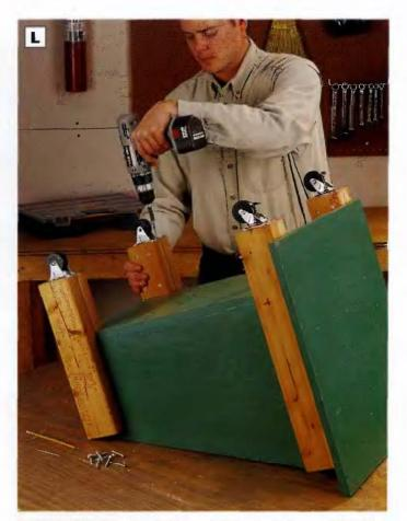
PHOTO L: Attach casters to the cart leg and cleat assemblles. We used swiveling locking casters on the front legs and fixed casters on the back. If you plan to fill the cart with dirt, be sure the casters are sturdy.
