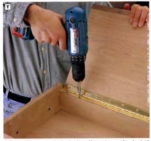
PHOTO T: Dry-fit the IId by attaching the piano hinge with one or two screws in each end and another in the middle. Remove the hinge, once you're satisfied that everything fits together, and reattach it after the finish is applied.
