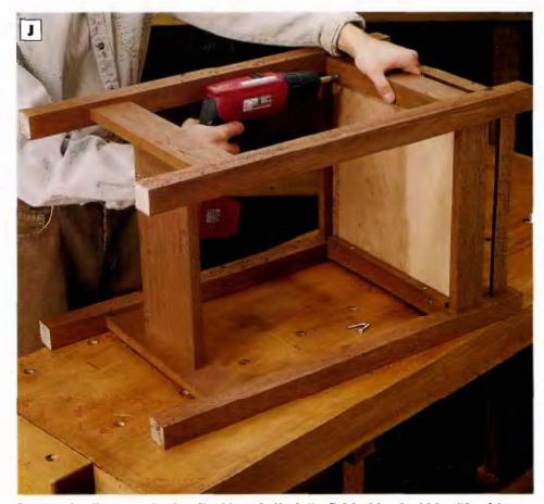
PHOTO J: Lay the plant stand on its side and attach the finished tray by driving #6  $\times$  1-in. screws up through the countersunk screw holes in the bottoms of the tray cleats.
