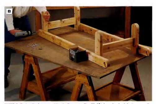
PHOTO B: Fasten the leg assemblles to the seat rails with  $2^{1}$ /2-In. galvanized deck screws. Be sure the foot rest notches on the seat rails face down on your worksurface when you fasten the legs to the rails. Check the leg assemblles with a square to be sure they are perpendicular to the rails before driving the screws.
