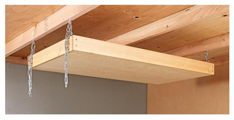
Connecting the snap links with the rafter-mounted eye bolts holds the tray closed. Both front corners of the tray, however, also have a short length of chain that's connected between the eye bolts with quick links. To access the tray, release the snap links and gently lower the tray until it's supported by the chains.
