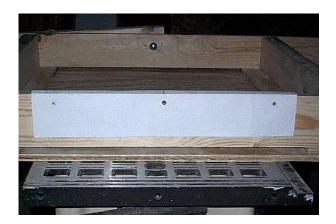
On the top edge of the Table Extension that will touch the saw table top, mark the center of the Table Extension; line up the center of the paper template to the center of the Table Extension; using the marks on the template, drill the three holes @ 3/16".
