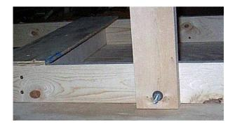
Select one,  $2 \times 4$  Support Leg; center it perpendicular on the outside edge of the extension; drill a 3/16" hole and connect the leg to the extension with a screw and wing nut (allow it to remain loose so it may be moved out of the way in the next step).
